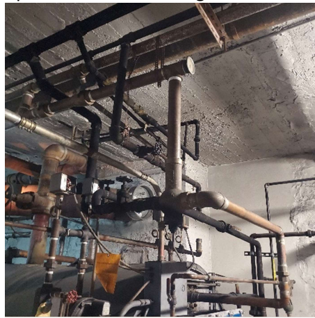
Figure 7.2.2 Mixing valves
