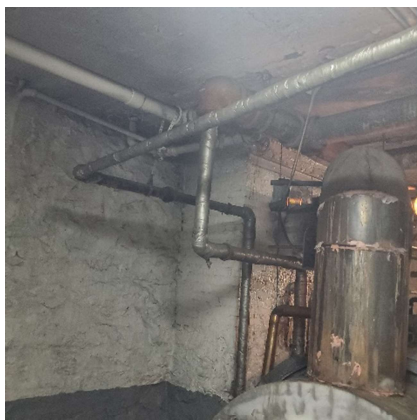
Figure 5.2.5 Condensate Return piping
