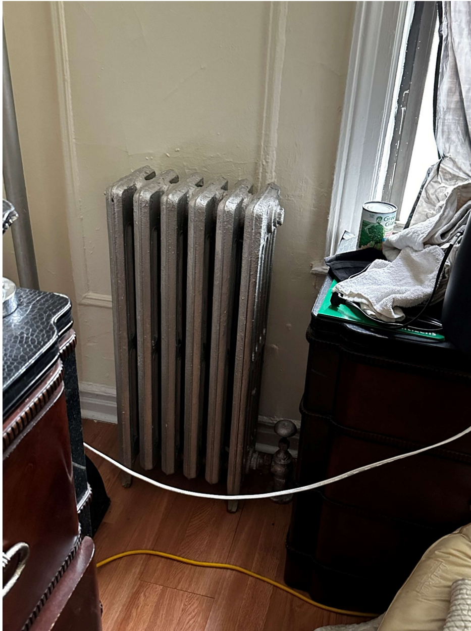
Fig. 8.5.1 Example of One pipe radiator @
