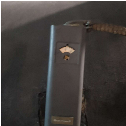
Figure 3.2.7 Boiler Aquastat
