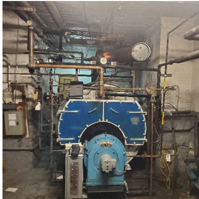
Figure 5.2.1 Steam Boiler & Piping Configuration
