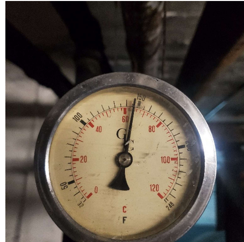
Figure 1.2.2 Domestic Hot Water Set Point
