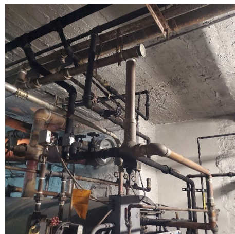
Figure 5.2.4 Mixing Valve for Domestic Hot Water Generation and piping
